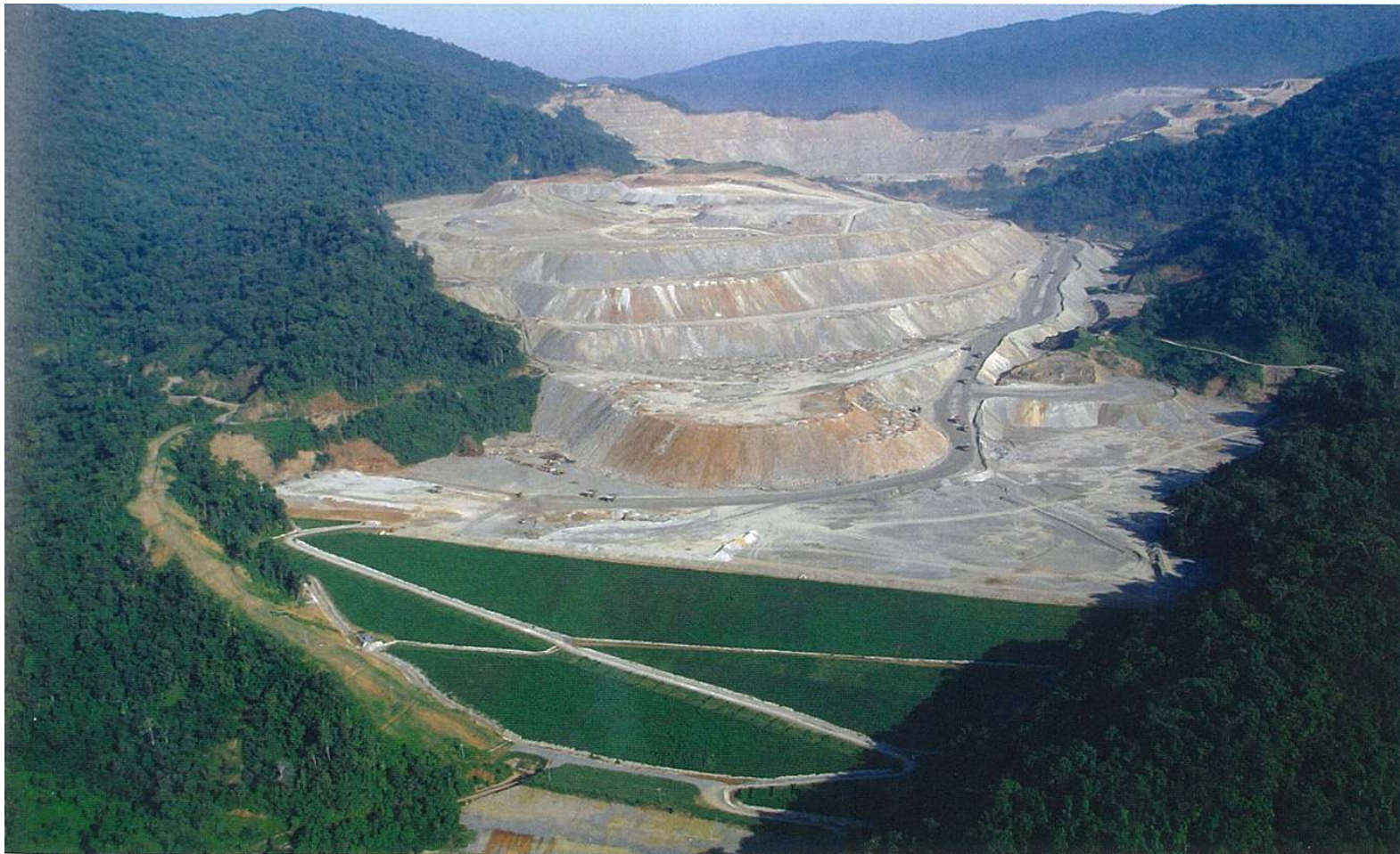
Concurrent reclamation of waste dump (Read and Stacey, 2009)
